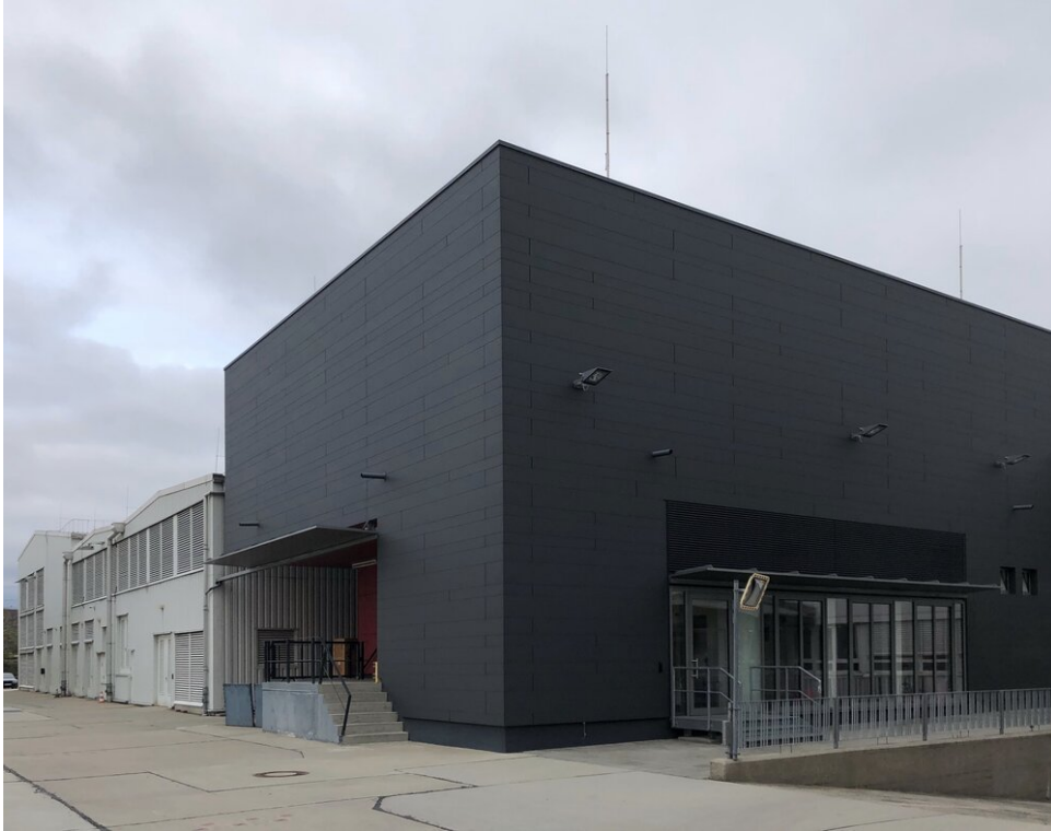
Datacenter in Frankfurt
